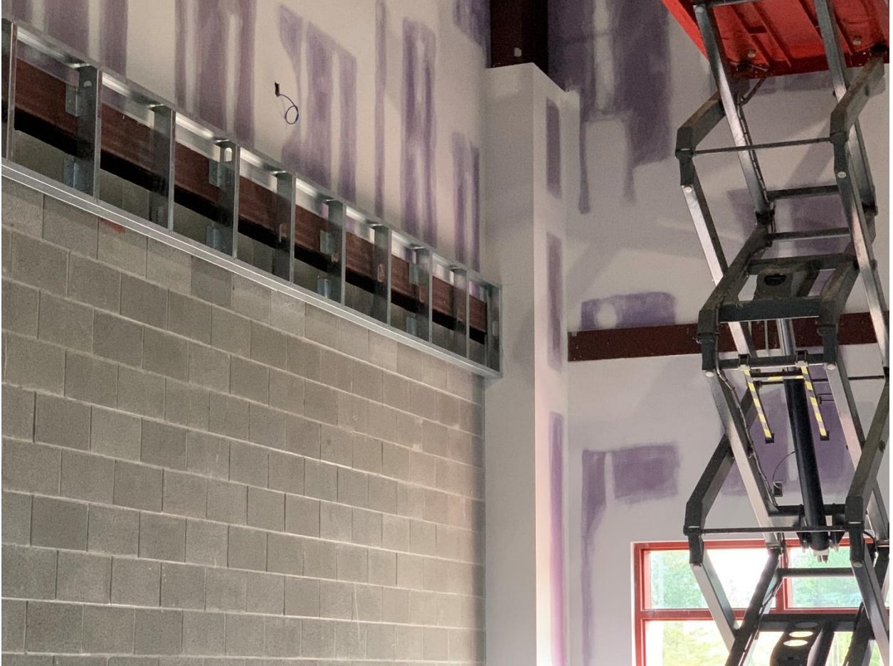
The weight room does not have a finished ceiling. The red conduit is for the fire alarm system and is located in the weight room.
